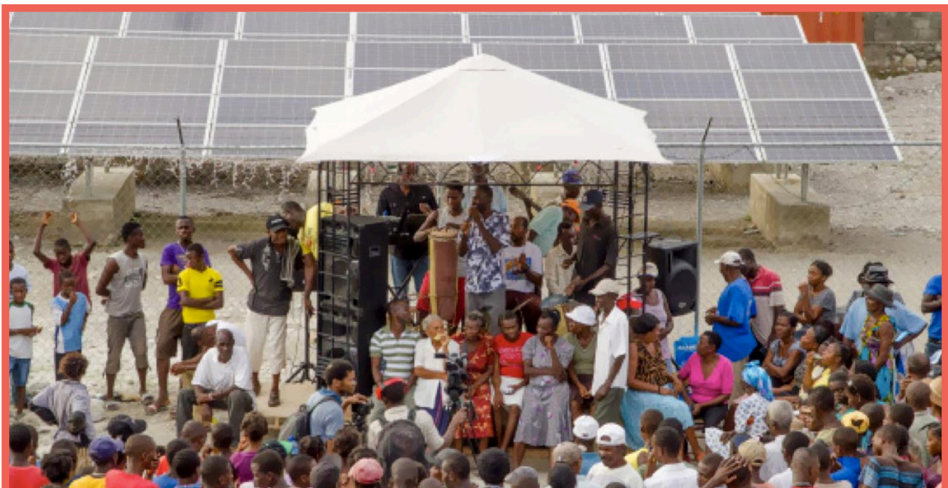
In 2015, Les Anglais, Haiti inaugurated its first solar-powered microgrid, a small step in the diversification away from hydrocarbon-fired electricity.
